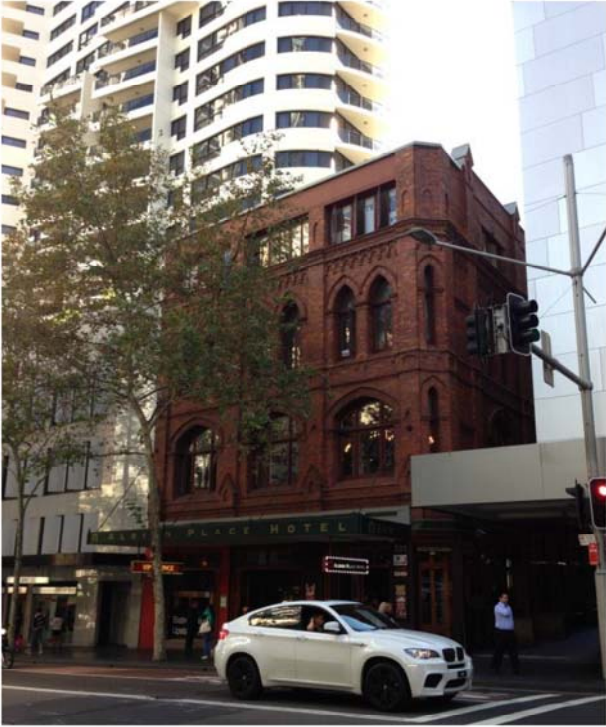
PICTURE 9 – THE ALBION HOTEL – THE FORMER 'VINE HOUSE' - 531-535 GEORGE STREET - ITEM #1795. THE MERITON RESIDENTIAL TOWER IS VISIBLE BEHIND
