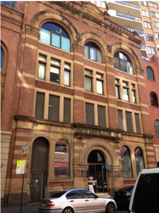
PICTURE 11 – THE FORMER WAREHOUSE FAÇADE - 533-539 KENT STREET - ITEM #1836
